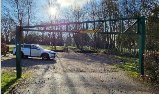
Figure 2 – John Pears car park entrance
